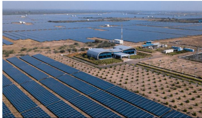
Figure 7: Adani Green Energy Plant
